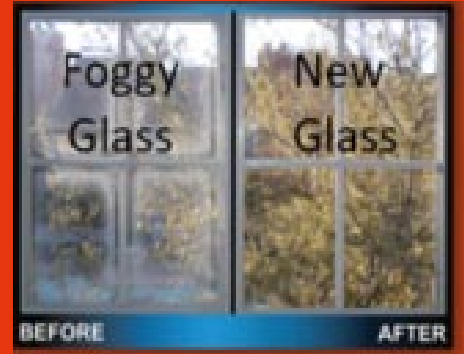
Foggy Glass Replacement
